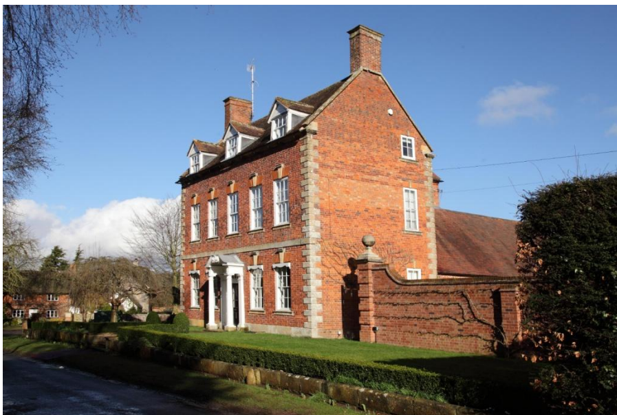
Figure 4 - Cleavers - Grade II* listed building circa 1740 (in the Conservation Area)
